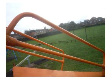
The step access fails entrapment requirements (at steps – distance should not be between 89 and 230mm) – Recommend monitor – Low risk.
