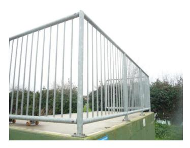
Gap between platform and lower edge of barrier should be 60mm (currently 100mm) – Recommend monitor only - Low risk.
