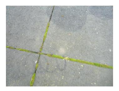
Trip zones found at edge of surface – Recommend build up ground levels to remove trip hazard – Low to Medium risk.
